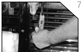
7. Disconnect both electrical plugs and install weather cover on both ends.
